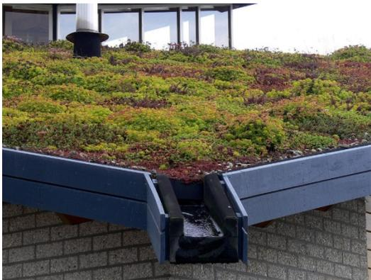
roofs can reduce the amount of water that accumulates in the storm drains, which results in easier manage storm water.
