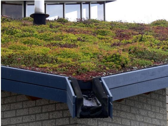
**A green roof on the Central Plaza performance stage could be beneficial for storm water management.** Placing green roofs on the wings of a performance stage in Central Plaza will provide benefits in storm water management and provide an artistic look to the performance stage.
