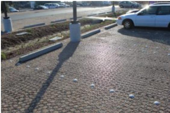
Permeable poured concrete and asphalt are made of a coarse aggregate that is coated in mortar and cement paste. This creates a structure that allows water to filter through to the ground surface. There are some issues
