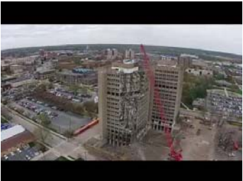
Demolition of Statesman Towers
