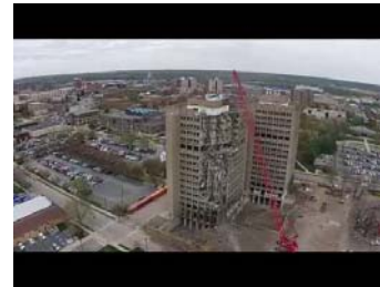
Demolition of Statesman Towers
