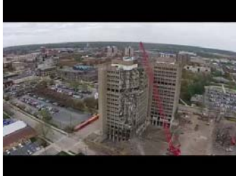
Demolition of Statesman Towers
